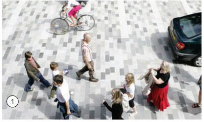
Paving Type 1: Feature Junction and Main Street Paving Granite paving units: 200 x 300 mm Colours: Ratio of grey tones - akin to New Road, Brighton
